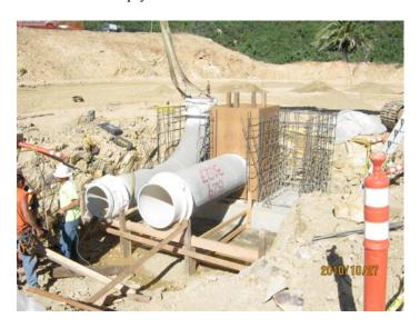
Excavation for both sumps was completed. Rebar and forms were received and rebar structures were built for both sumps, along with the core boxes to be place in each. As of the end of the month, concrete had been poured in the floor sump for the south tank. Upcoming work should include commencement of tank construction with fabricating rebar and pouring the concrete bottom slab. Please visit the following web links for a running discussion and diagrams for this project:
